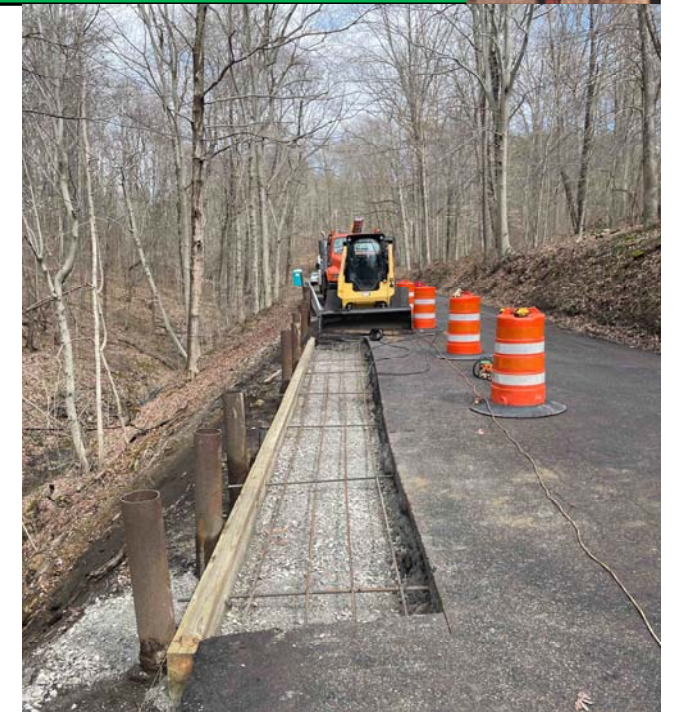
County Road 26 Base Repair Prepping for Pavement
