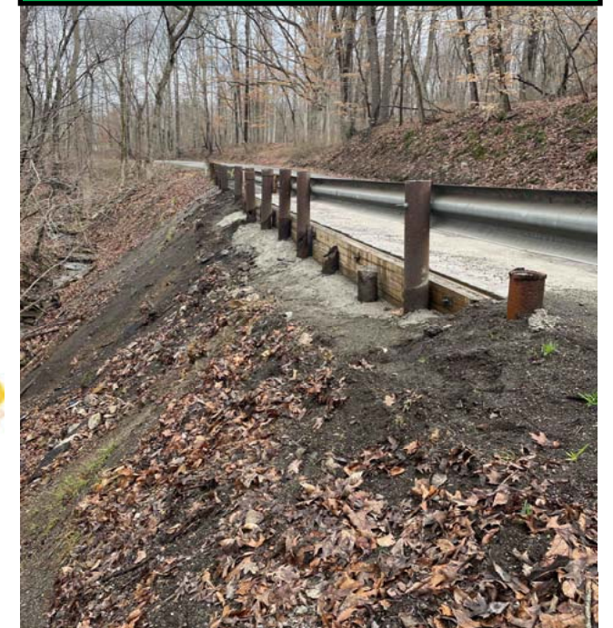
County Road 26 Base Repair Prepping for Pavement
