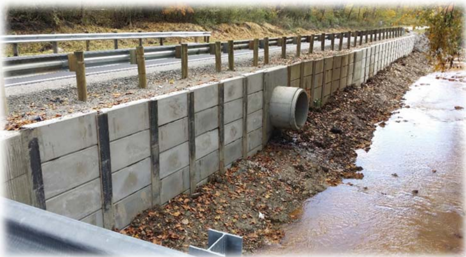
Willow Grove Road Retaining Wall After Repair
