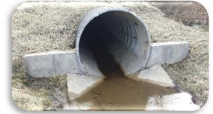
Oak View Rd Culvert repair
