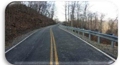
Fulton Hill Rd repair
