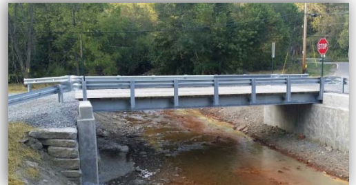
New Bridge following repairs on Wasniak Road Pultney Township T-281
