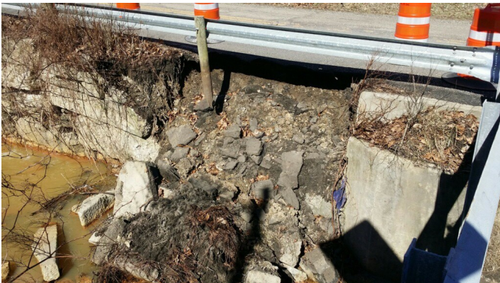
Wall collapse on County Road 2 Deep Run.
