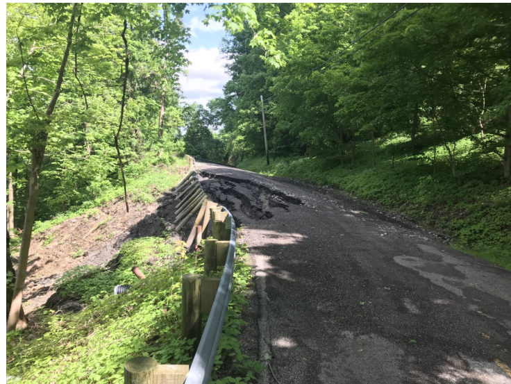
County Road 42 Fulton Hill embankment failure.
