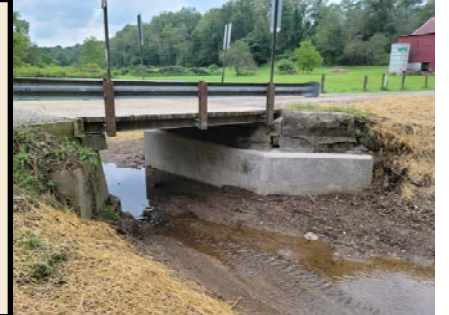
Somerset Twp T-39 School House Road
