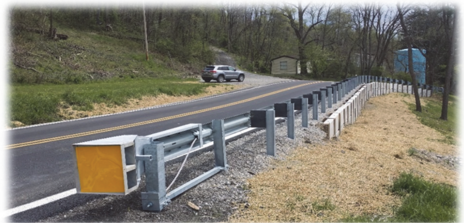
CR-20 – Blaine-Chermont Road Slip Repair
