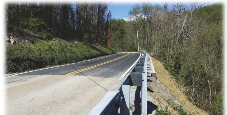
CR-102 – Mt. Olivett Road Slip Repair
