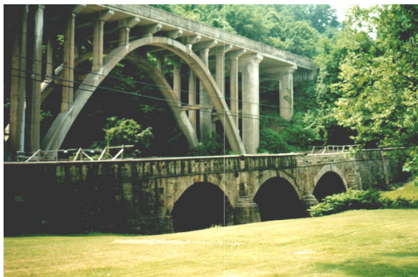
Historic Blaine Bridge 1996
