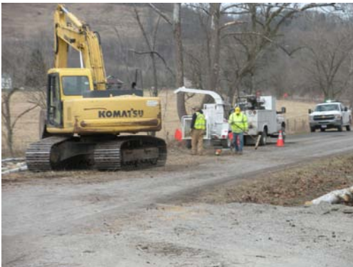
Clearing trees on County Road 10 bridge project.
