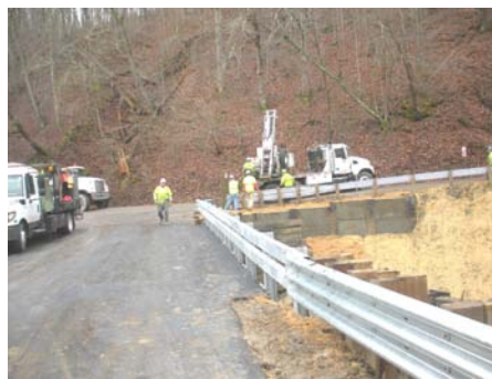
County Road 54 Pipe Creek
