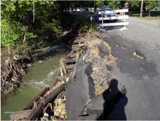
County Road 2, Deep Run
