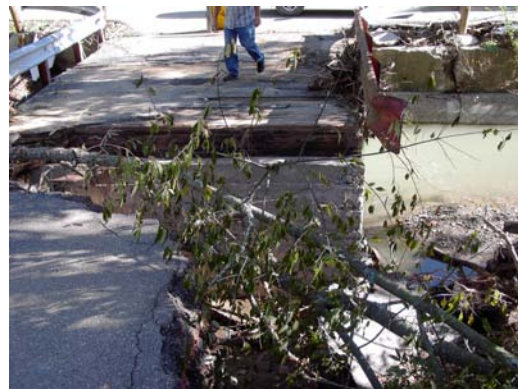
Pease Township 641 Bridge
