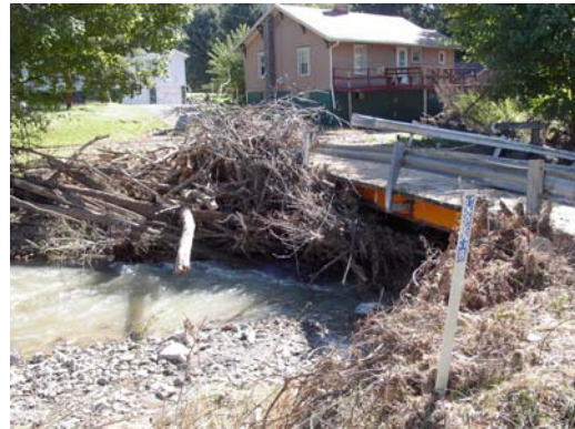
Richland Township 1249 Bridge
