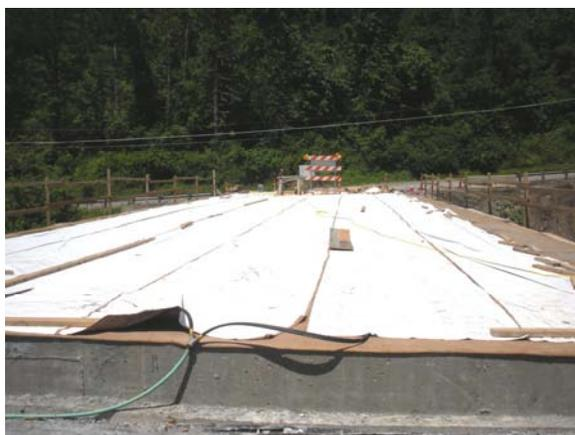
Shown on the left is the new concrete deck curing on the County Road 4, Sand Hill bridge replacement project.
