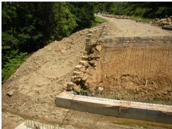
Work is progressing on the renovations of 2 historic stone arch bridges located on Union Township Road 814 and County Road 40B. Shown at left is poured footers on County Road 40B.
