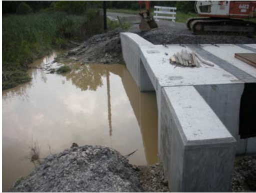
Co. Rd. 98 Badgersburg Road bridge replacement nearing completion.
