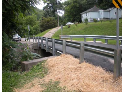
Pultney Township 325 Indian Run bridge replacement completed.
