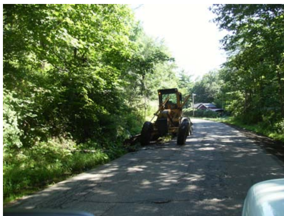
Ditching on County Road 5, Crescent 250.
