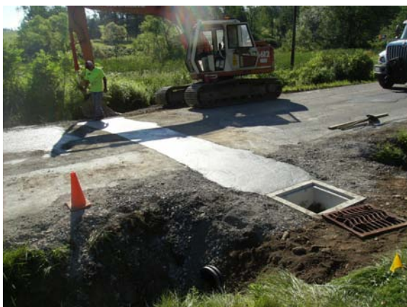
Culvert replacement on County Road 82, Airport Road.
