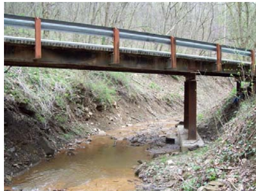
The steel girder bridge pictured below was replaced with a 3 sided aluminum box culvert by the Ohio Department of Natural Resources.
