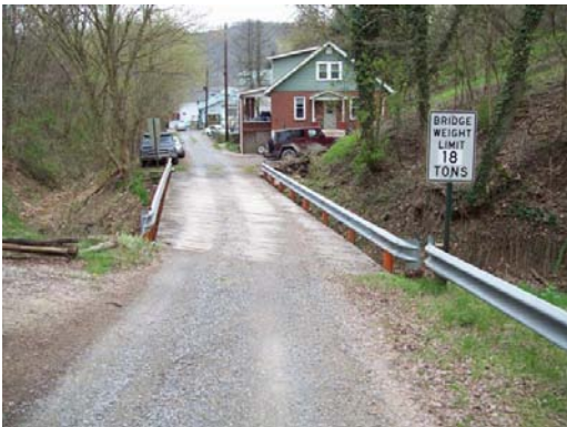
The steel girder bridge pictured below was replaced with a 3 sided aluminum box culvert by the Ohio Department of Natural Resources.
