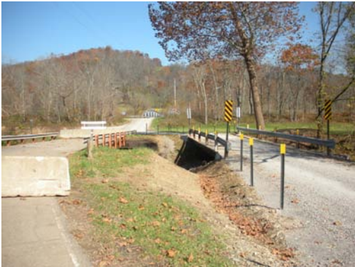
County Road 5, Clover Ridge, temporary bridge in place.
