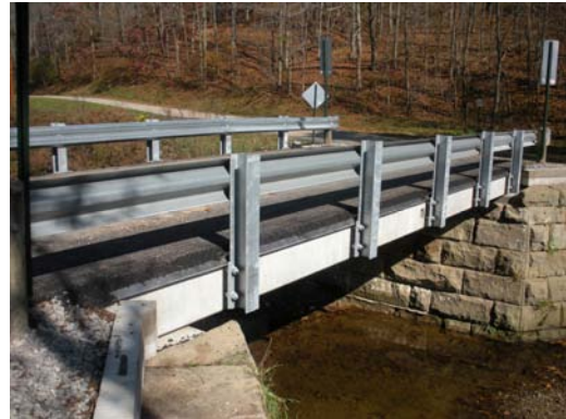
Wayne Township T-87, Mayhugh Road, bridge replacement.
