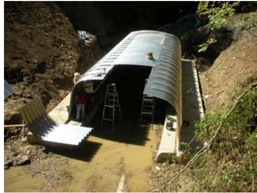
The steel girder bridge pictured below was replaced with a 3 sided aluminum box culvert by the Ohio Department of Natural Resources.
