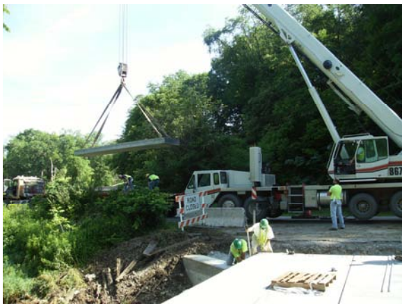
These photos show the concrete beams being set on Flushing Township Road 597, located near Holloway. The beams were supplied by Carr Concrete. The crane & operators were from Nemo Hauling Rigging & Crane.
