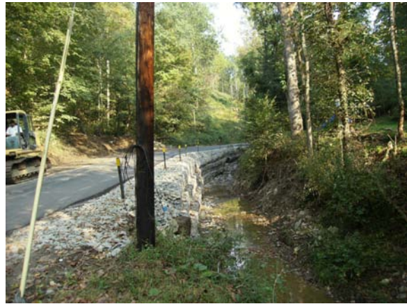
The slip repair project of County Road 5, Glencoe St. Clairsville Road has been completed. The area was damaged during the heavy spring rains that occurred throughout May and early June of this year.
