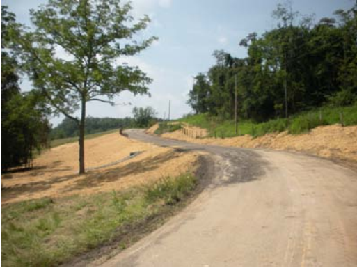
Completed road slip repair on County Road 56 - 13.60.
