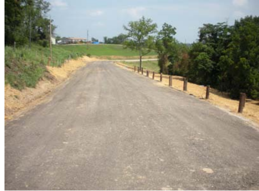
Completed road slip repair on County Road 56 - 11.62.
