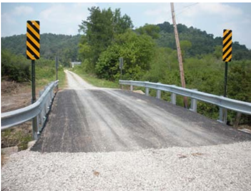
Flushing Township Road 597 bridge replacement project.
