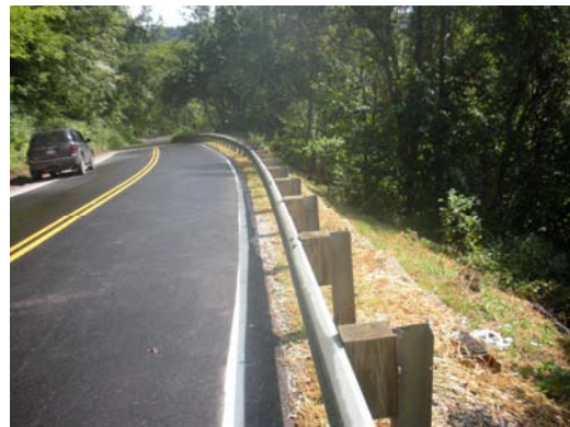
This piling project on County Road 4, St. Clairsville Barton Road was administered by ODOT / FHWA..
