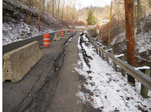
County Road 16, Nixon Run, piling project started this week.
