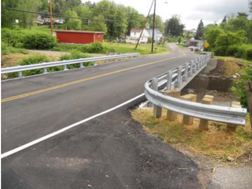
County Road 48, Wegee, first bridge completed on Project 10-4.
