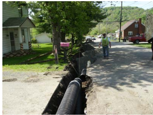
County Road 30, Dixon Hill. Road crews recently finished this culvert project near the intersection of State Route 149.
