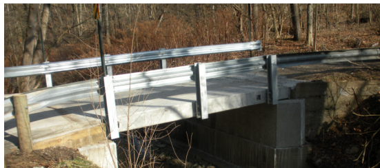
Recently completed bridge replacement on Pease T-471.
