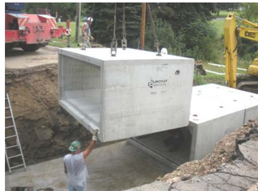
The bridge crew recently completed this concrete box culvert project on County Road 26 in the Village of Bethesda.
