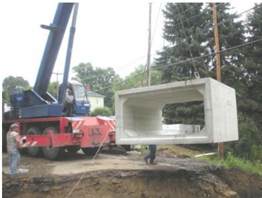
The bridge crew recently completed this concrete box culvert project on County Road 26 in the Village of Bethesda.
