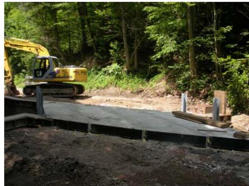
The bridge crew set the concrete box beams on the Richland Township Tar Run Bridge on June 1.
