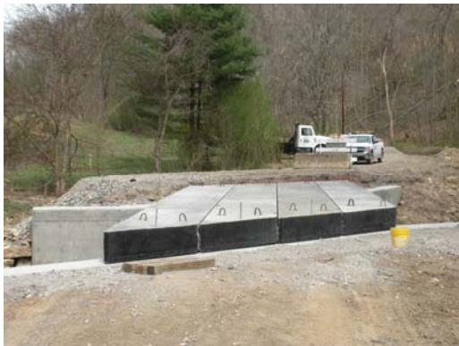
Two bridge replacements are nearly complete on Richland Township Road 284, Bull Run. Both bridges were force account projects with the concrete beams being supplied by Carr Concrete.
