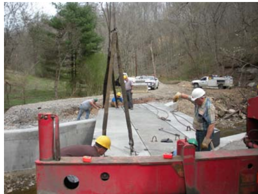
Two bridge replacements are nearly complete on Richland Township Road 284, Bull Run. Both bridges were force account projects with the concrete beams being supplied by Carr Concrete.
