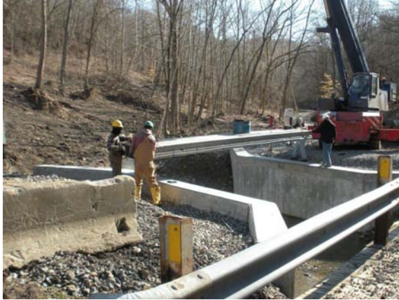
Concrete box beams being set on Richland Township Road T-284, Bull Run Road.
