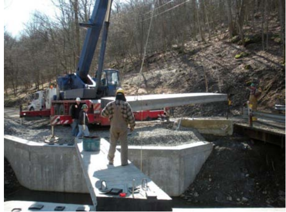
Concrete box beams being set on Richland Township Road T-284, Bull Run Road.
